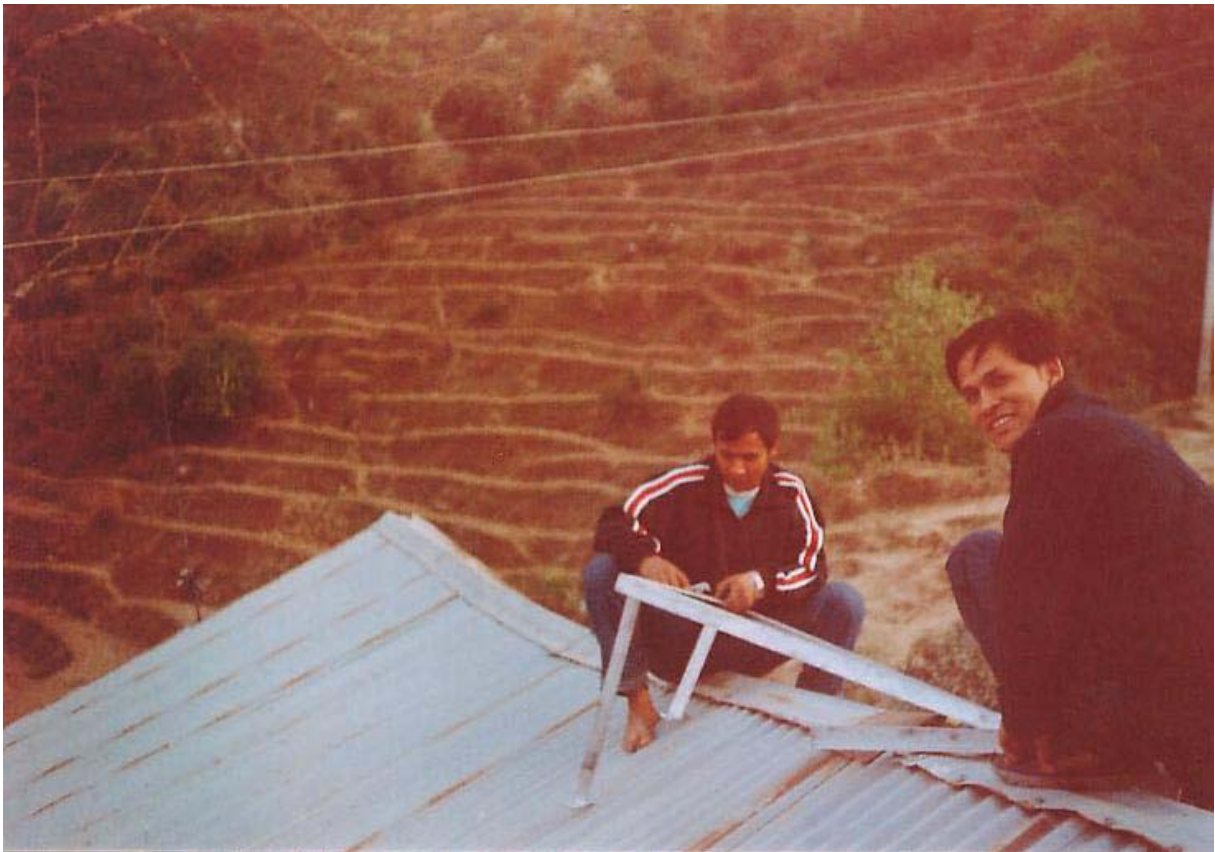
Fig 1: Lasersun Technicians installing the solar panels
