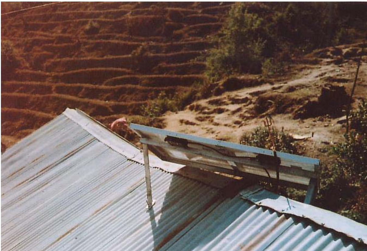
Fig 2: Installation of Solar Panel
