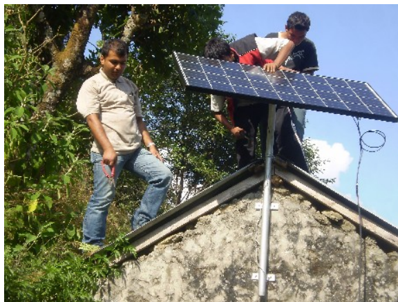
Fig. 1: Installation of the Solar Array on the roof
