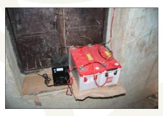
The batteries are standing to the metal windowcloser. Because the sun burns onto the metal plate these where very hot, to hot to touch.
