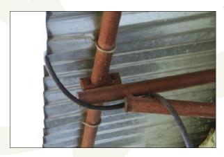
The isolation between the cable and the construction is to thin. If lightning would occur then it will electrify the metal construction.
