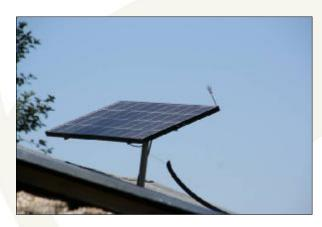
For a good lightning arrestor system you need a metal pole with a diameter of at least 1cm standing next to the solar panel, about 1 meter higher then the highest point of the solar system. This 'fork' is too small.
