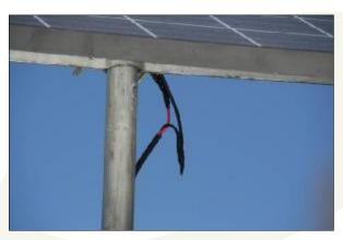
The connections of the wiring is not acceptable. The engineers connected them by hand and put tape on it, inside the building and outside. This tape will get loose within a few months with blank wires as result.
