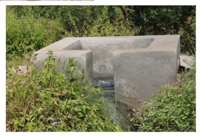
3 distribution chambers built from where the irrigation water is diverted to the fields. 8.90 hectares of farmland is expected to have access to sufficient irrigation water even during the dry season. The farms are irrigated turn by turn, where each farmer gets sufficient water according to the need and the area of farmland.
