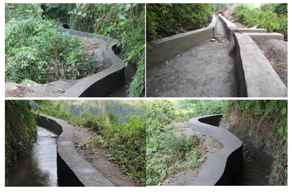
Newly constructed canal - PCC (Plain Concrete Cement) on the base, stone walls cemented on both sides. With proper care this canals will provide irrigation water for a long time.
