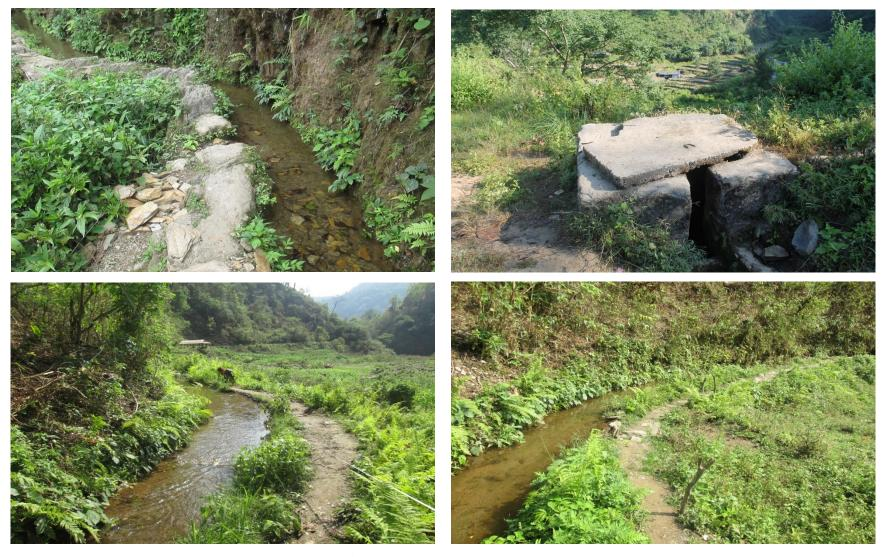
The crude irrigation canals had many flaws; water flow was stunted, leakages in numerous places, and technically very poor in design. Water loss was high and never sufficient for the fields, thus, resulting in poor crop yield.
