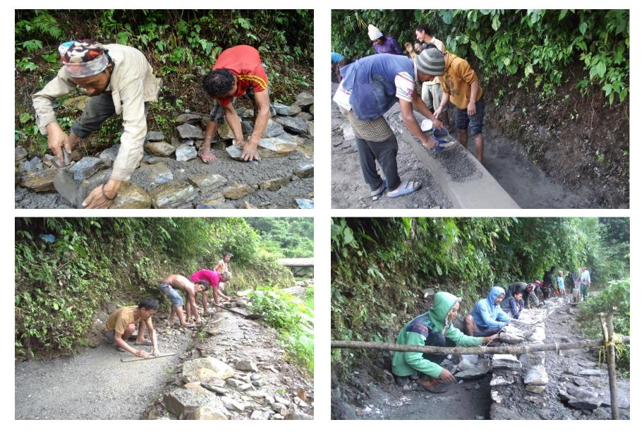
1,532 Man Days were contributed by the community and 492 Man Days were resourced for skilled labors. Masons working during the construction of cemented canal. 1,100 meters of canal were reinforced with cement and made sturdy.
