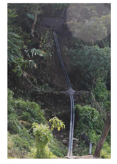
130 meters of HDPE pipes are used for the crossing. This made it possible to provide access to irrigation water to 3 hectares of farmland for Banauti village.
