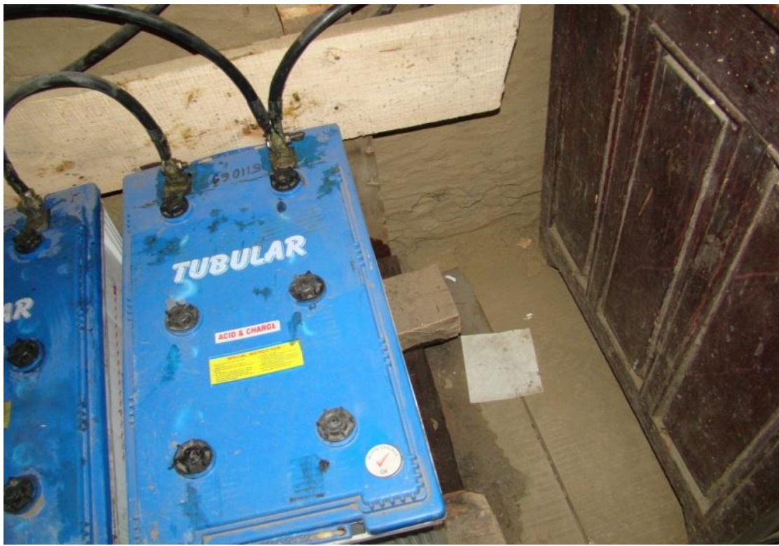
Fig.2: Tubular Battery Placed On Wooden Frame
