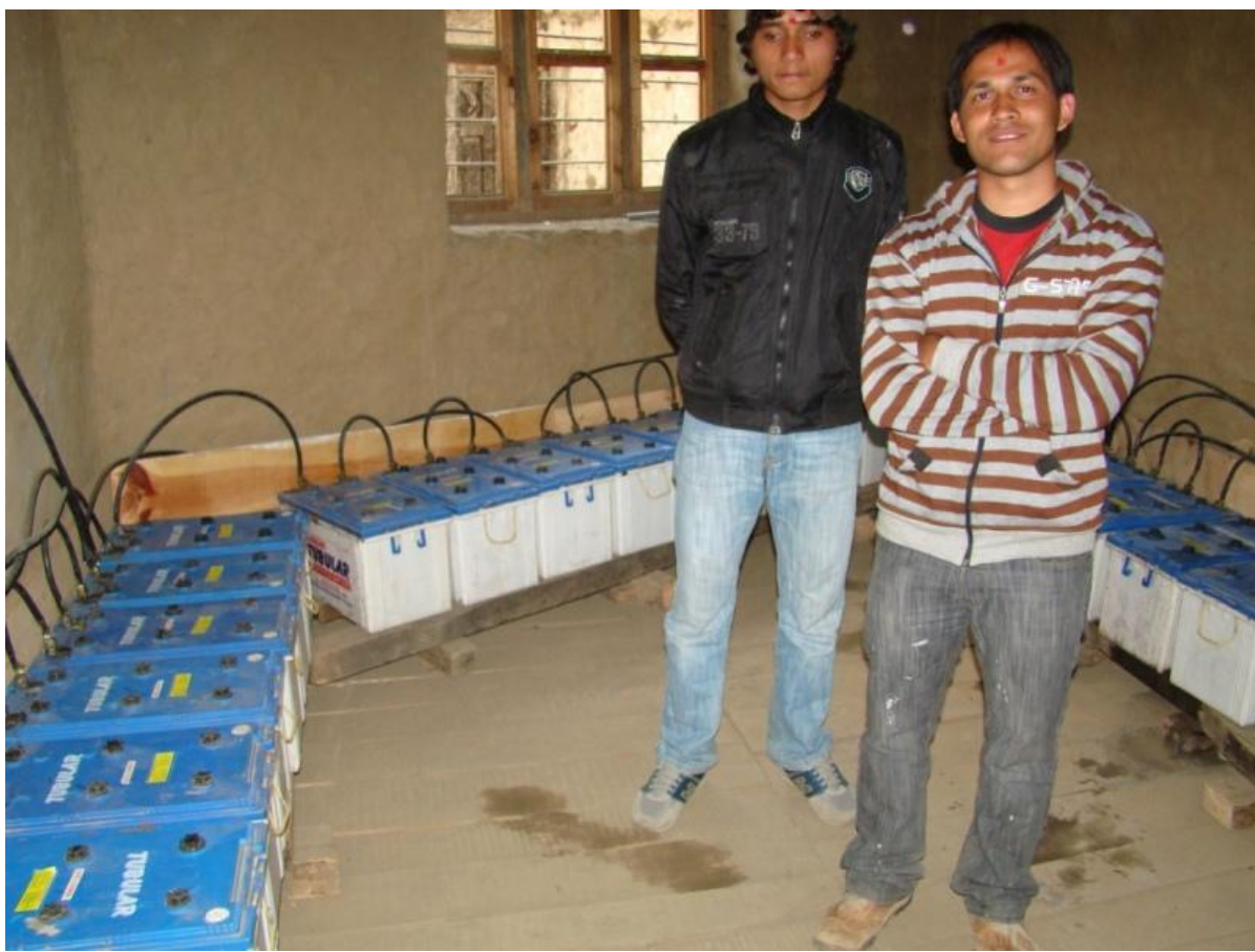
Fig.3: Battery Bank Of 32 Batteries
