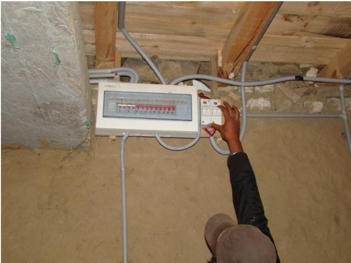
Fig.5: Connection Of AC Distribution Box And Breakers
