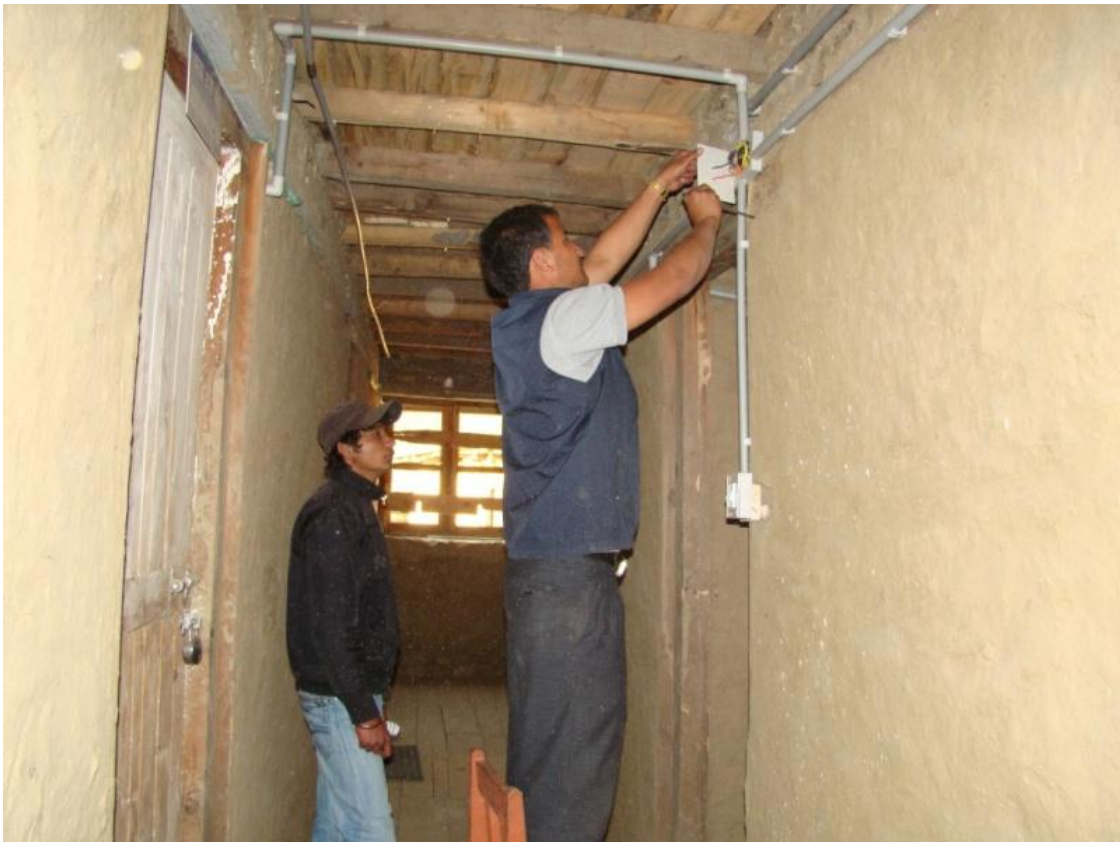
Fig.6: Lasersun Staff Performing Conduit Wiring
